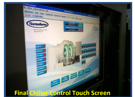
Chiller Controls After, in NEMA 4 Cabinet
